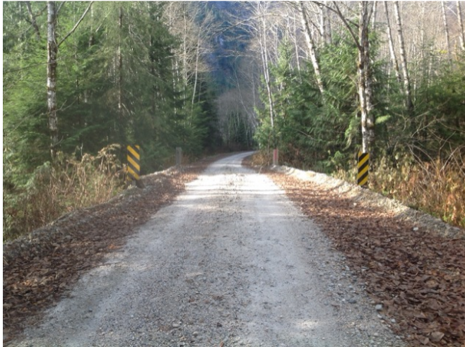
Approach from Left Bank when facing downstream
